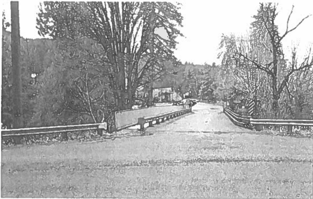
Subject Entry / Bridge over Little Elk Creek
